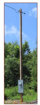
United's crew will install the service entrance (meter loop) for members also having a meter pole installed by the co-op. The total price is \$1.325.44. for the meter loop and pole installation. The meter loop consists of a 100 or 200 AMP meter base/disconnect panel (must be the same as main breaker in the structure). weatherhead. entrance cable. ground rods, ground fault receptacle
